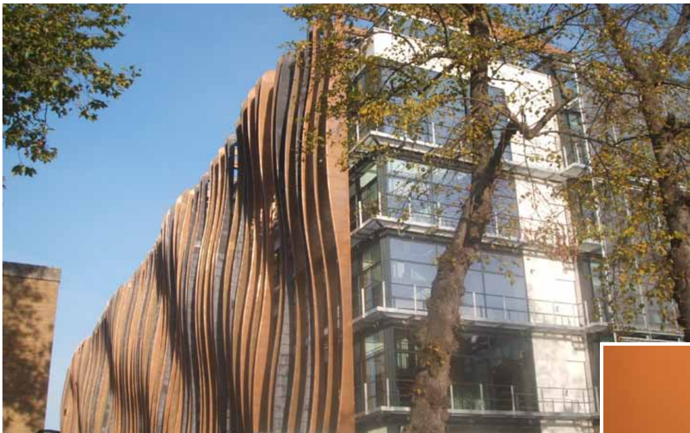
Vertical solar shading fins, each clad in either Nordic Bronze, Nordic Brass or Nordic Brown™. Holland Park School, London; Architects: Aedas.
